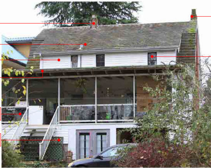
B. VIEW OF THE NORTH REAR OF THE HERITAGE HOUSE
