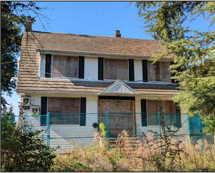
Fig. 1: Front view of 13761 Grosvenor Road, 2025. (Source: Cummer)
