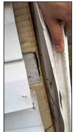
Figs. 15a and 15b: (Left) View of the exploratory opening revealing the extant wood siding, 2026. (Right) View of the corner detailing, showing it was originally likely mitred rather than with corner boards. (Source: Dhaliwal)
