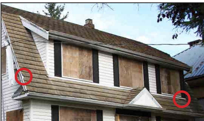
Fig. 11a (top right): Rear view of 13761 Grosvenor Road, 2024, showing the condition of the roof, in particular the moss growth (outlined in red). (Source: Luxton)
