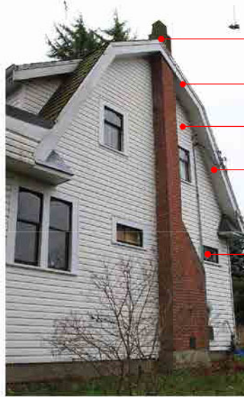
D. VIEW OF THE WESTERN SIDE OF THE HERITAGE HOUSE
