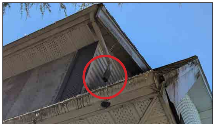
Fig. 11a (top right): Rear view of 13761 Grosvenor Road, 2024, showing the condition of the roof, in particular the moss growth (outlined in red). (Source: Luxton)
