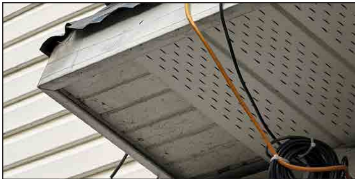
Figs. 14a and 14b: (Top) View of some of the visible wood elements, 2026, including fascia and soffits. (Bottom) Closer view of the original closed wood soffits beneath the vinyl. (Source: Dhaliwal)
