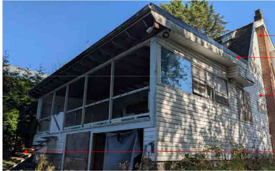
C. VIEW OF THE WESTERN SIDE OF THE HERITAGE HOUSE
