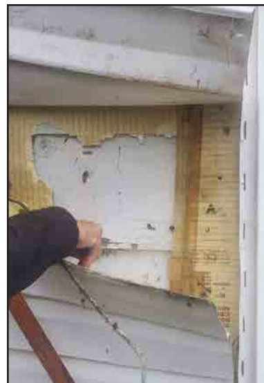
Figs. 15a and 15b: (Left) View of the exploratory opening revealing the extant wood siding, 2026. (Right) View of the corner detailing, showing it was originally likely mitred rather than with corner boards. (Source: Dhaliwal)
